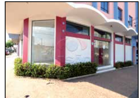
58303 - Centro - At 100 M 2 - Ac 76 M 2 - 2 Salas / Coz / Wc / R$ 2.500,00
